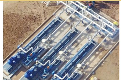
To satisfy the operator's technical specifications, Valiant was tasked with providing a horizontal pumping system (HPS) configuration capable of transferring 7,500 barrels of fluid per day at a discharge pressure of 2,264 psi, as well as supplying ancillary components required for the system such as pipe sections, check valves, and globe valves.
